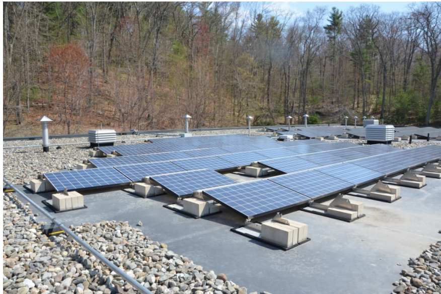
PV 1 on the plant's roof, secured in place by cinder blocks. The stones surrounding the array, as well as the weight of the array itself, hold down the roof's rubber membrane.
