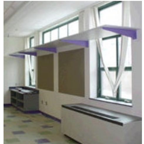
This lightshelf is part of the energy efficient design at the new Capuano School, the first Leadership in Energy and Environmental Design (LEED) registered public school in New England. (Somerville CAP, 2003)
