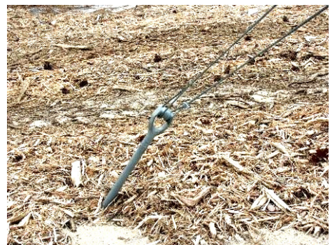
An anchor, installed, with 2 guy wires attached
