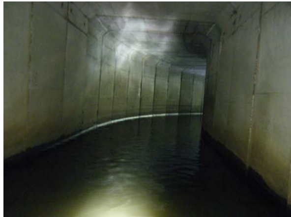
Mill Brook conduit extension under Worcester downtown.
